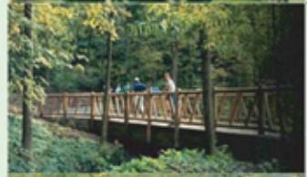
Trail Example Bridge
